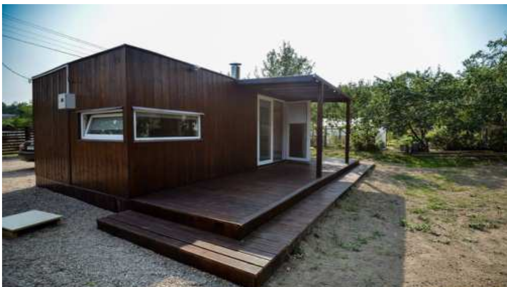
Fig. 2. Container house built in Minsk region
