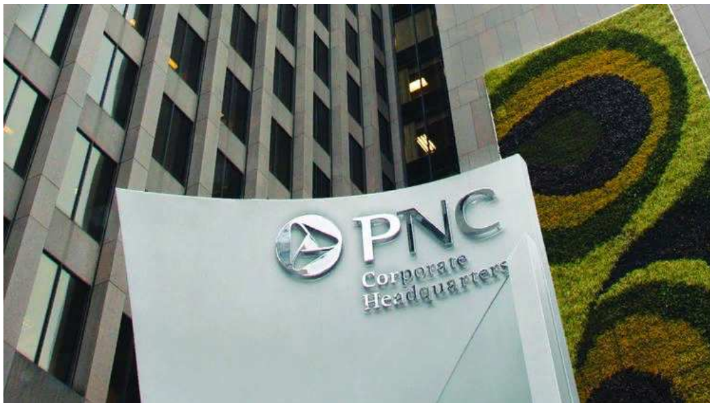
Figure 2. – Modular system of containers. One PNC Plaza in Pittsburgh
