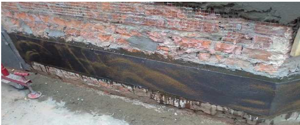
Figure 3. – Strengthening of brick walls with a tape of carbon fibers
