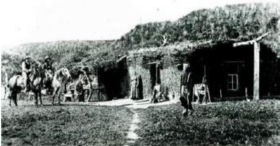
A Nebraska homestead in the late 19 th century. The house is made of sod bricks as the treeless plains supplied no lumber. The arrival of a stranger was a welcome break in the monotony of daily life
