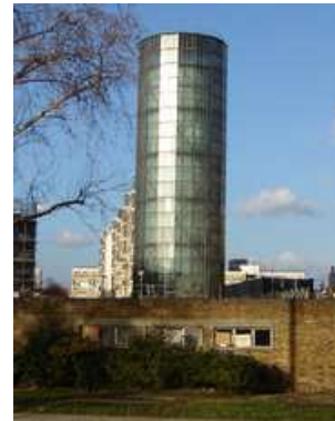
District heating accumulator tower in London. This plant use waste water piped from Power Station on the River Thames. (January2006)
