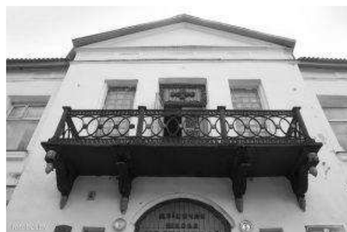
Figure 2. – Balcony of the second floor
