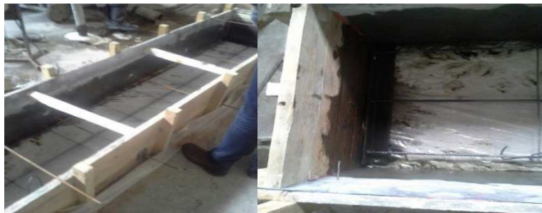
Figure 2.– A photo of the reinforcing grid laid in a timbering
