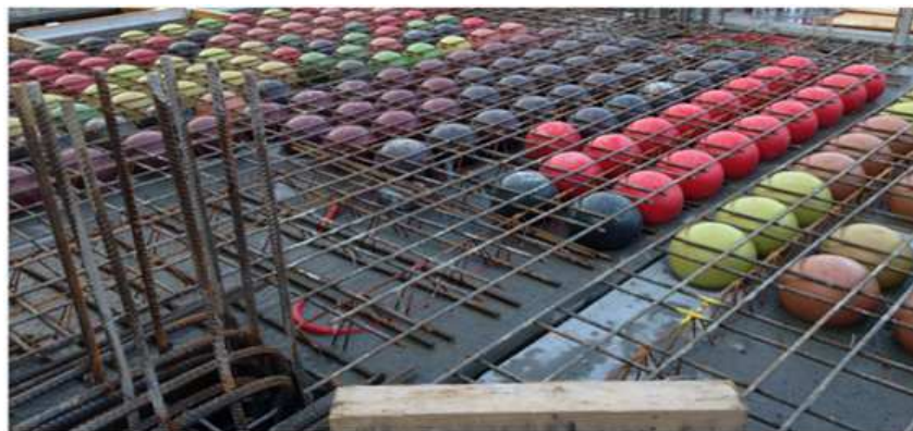
Figure 2. – The device is light weight concrete slab by bubble deck technology
