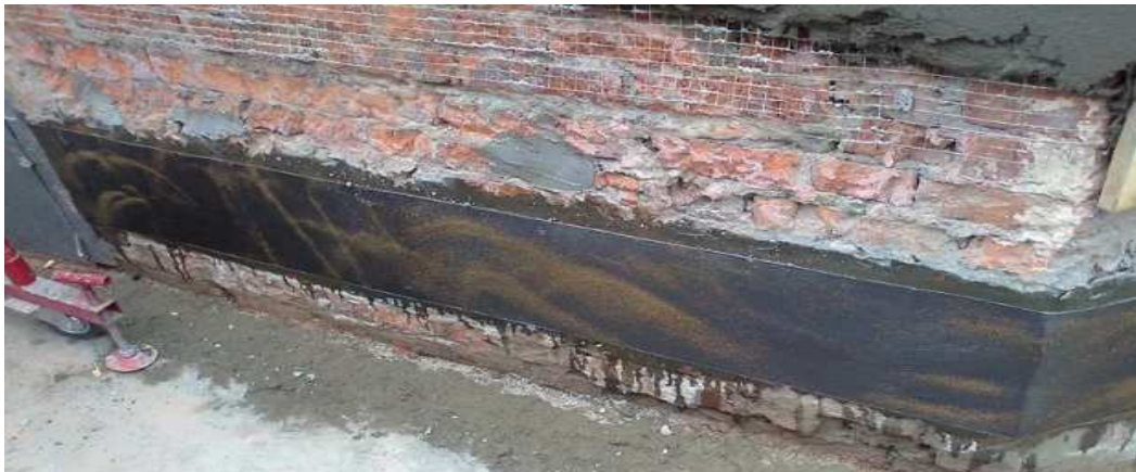
Figure 3. – Strengthening of brick walls with a tape of carbon fibers
