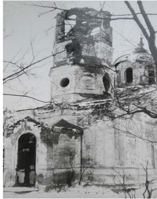
Fig. 2. The Church of the Resurrection before restoration
