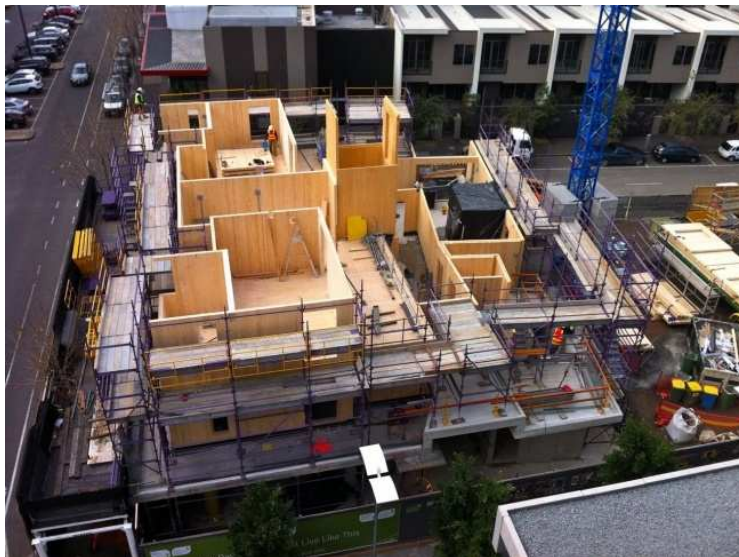
Fig. 2. Construction of a residential building Forté in Melbourne
