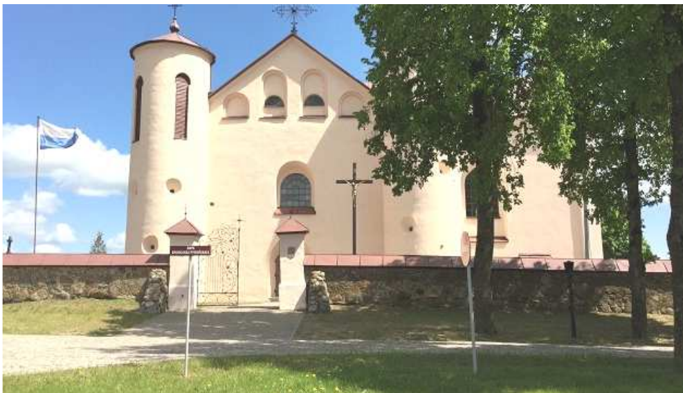
Fig. 1. St. John the Baptist Catholic church
